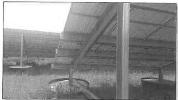
Figure 2. Fixed Axis Solar PV Array on a ballasted concrete foundation at the Town of Beacon Landfill, NY.
