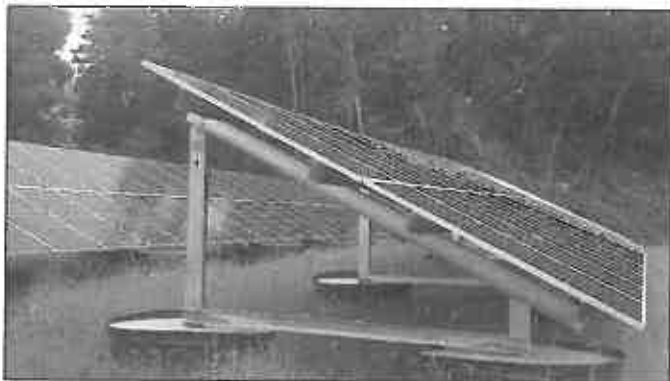
Figure 2. Fixed Axis Solar PV Array on a ballasted concrete foundation at the Town of Beacon Landfill, NY.
