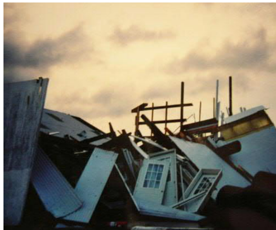
Photo 3a. 3 - Tornado Damage at Wiley Brothers Lumber and Hardware Store, Route 40, Schaghticoke, 1998
