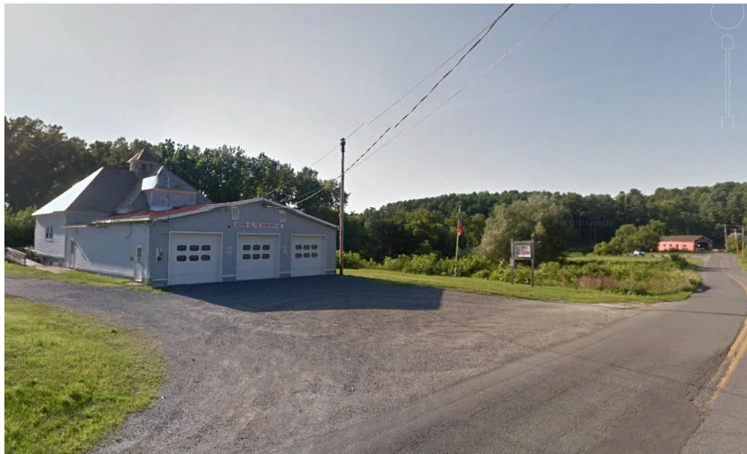
Photo 3c - 1. Photo, Buskirk Volunteer Fire Department. Looking north toward the Buskirk Covered Bridge. 2217 Buskirk West Hoosick Road Buskirk, New York 12028.
